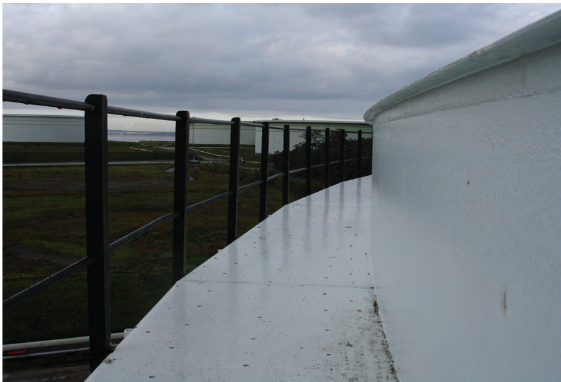
Figure 15 Top girder (walkway) on floating roof tank
